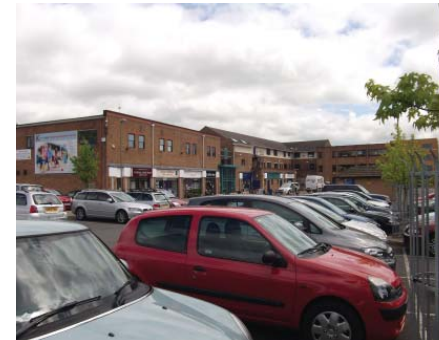
Figure 4.4 Surface car parking
