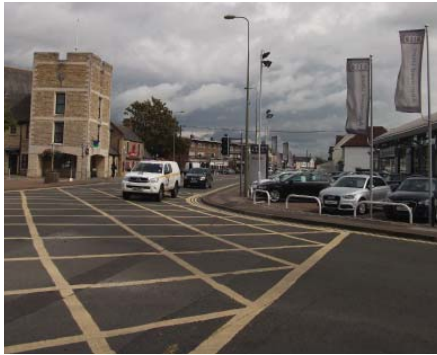
Figure 2.18 Box junction markings dominate the Oxford Road junction
