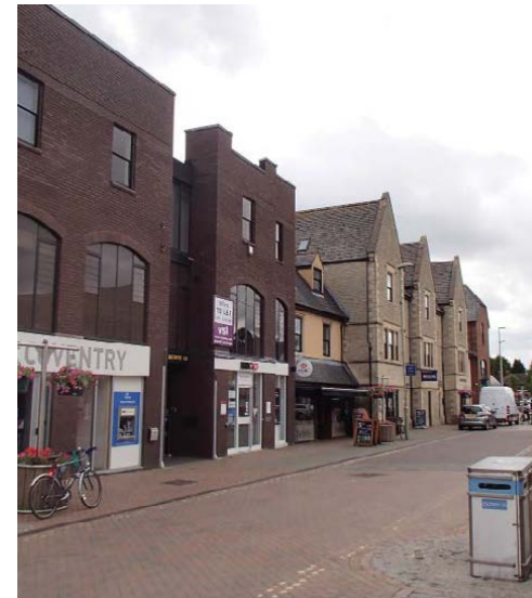
Figure 4.14 Three storey buildings on the southern side of High Street
