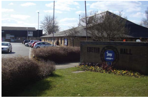
Figure 2.4 Village Centre - Exeter Close
