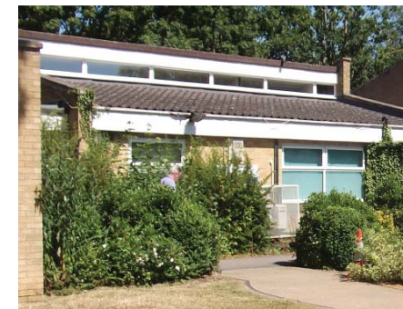
Figure 2.16 Health centre, Exeter Close
