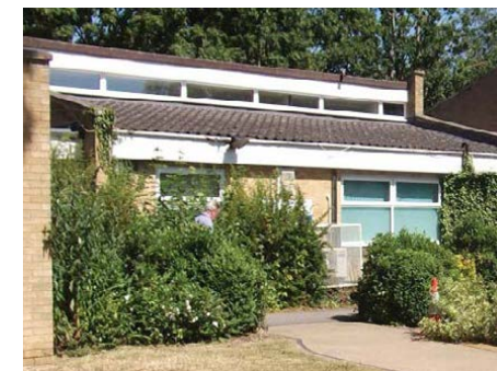
Figure 4.7 Health centre, Exeter Close
